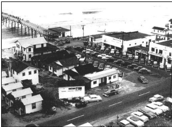
Pier Square before Hurricane Hazel in 1953
