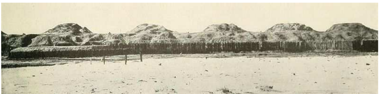
This is the 1864 view of Fort Fisher from the Atlantic Ocean. A 12 foot high timber fence was built along the beach.
