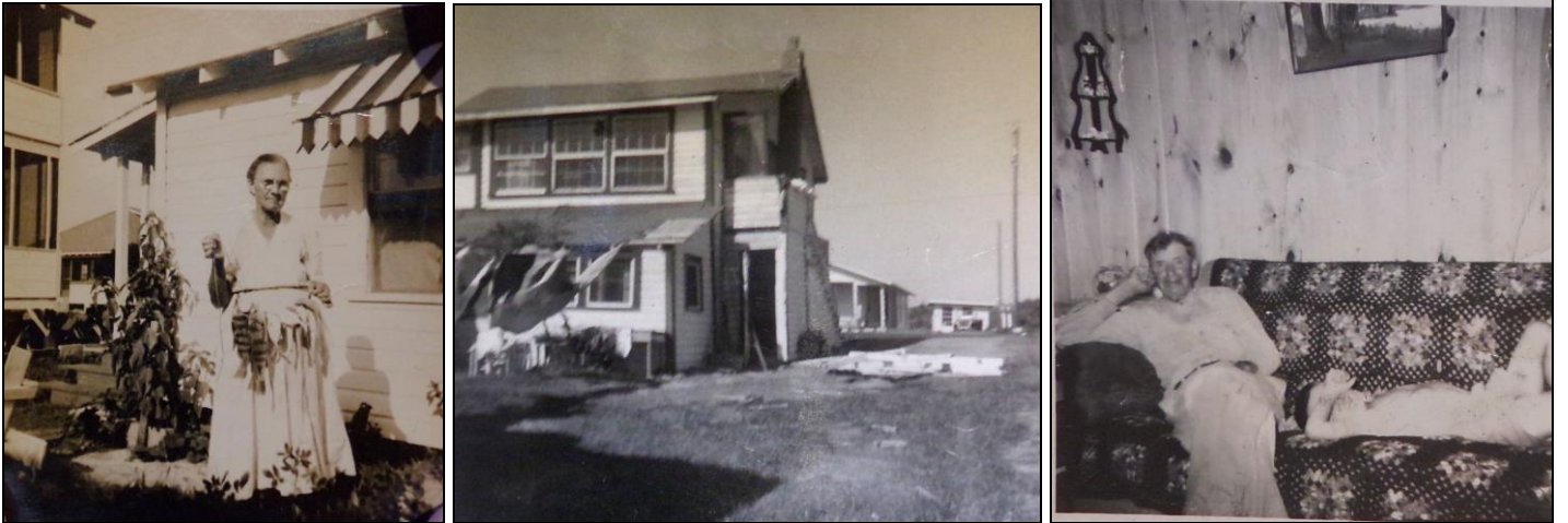
Grandma loved to fish. She extended the back of the house to make a larger room to rent and a back porch. She built a flat roof cottage between the house and the original cottage, and added a third cottage across the road in 1954, along with a storage building. Hurricane damage is shown in the center photo. On the right, Grandpa sits in the front living room with butch on the sofa in 1951. This is the only known photo of the inside of the house. I remember the knotty pine walls in all the rooms. Grandma made the cover on the couch, which appears again in the photo below, taken in front of the house.
