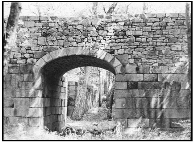
One of the stone bridges over the ten foot wide canal
